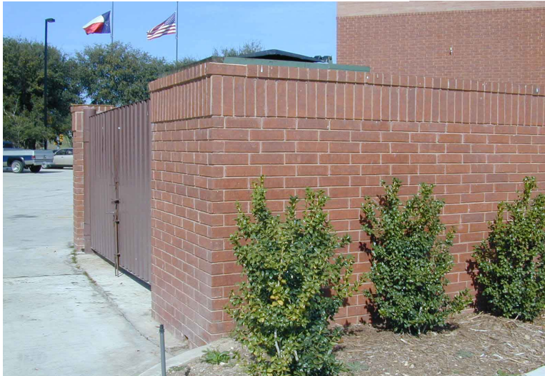
Figure 4.07.3. Example of Refuse Area Screening
